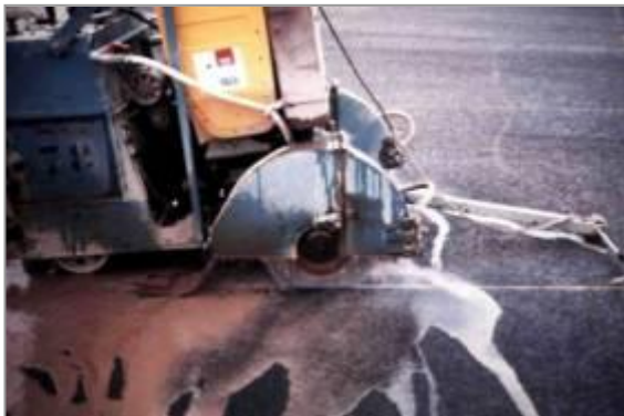
Figure 13 Cutting of the groove
