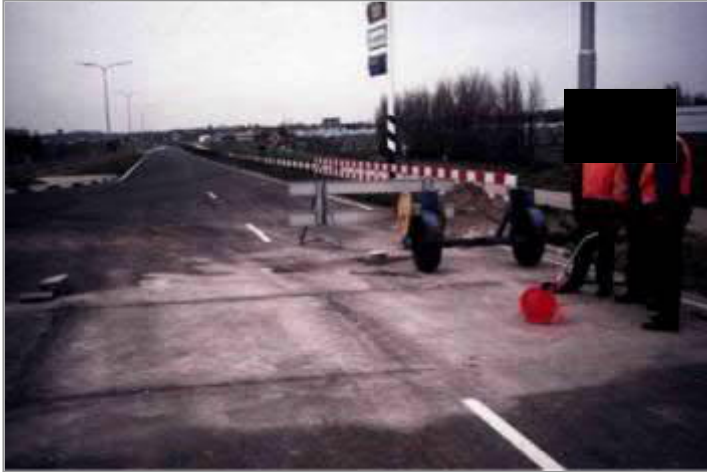
Figure 16 The grooves are cut
