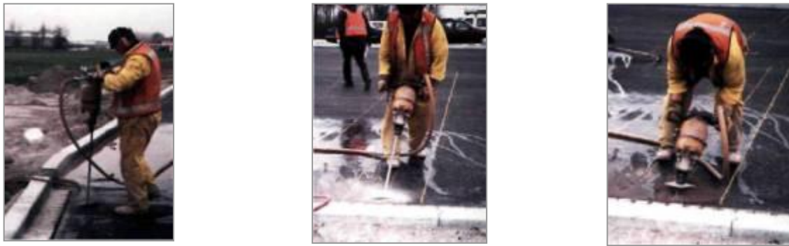
Figure 14 Groove cutting
