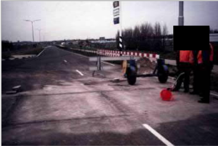
Figure 16 The grooves are cut
