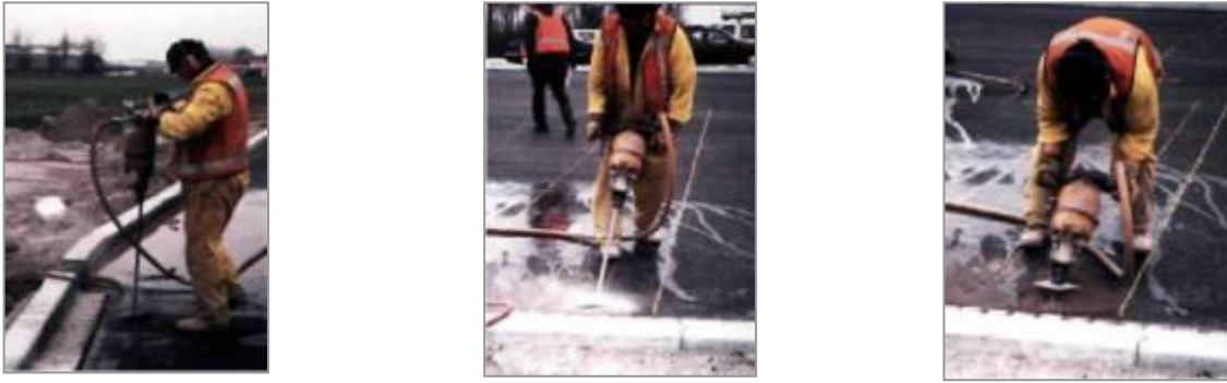
Figure 14 Groove cutting
